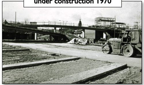
Wyvern footbridge under construction 1970
